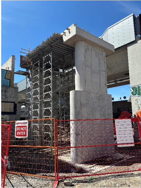
#1 Switchback ramp work (north landing) and south pedestrian bridge work
