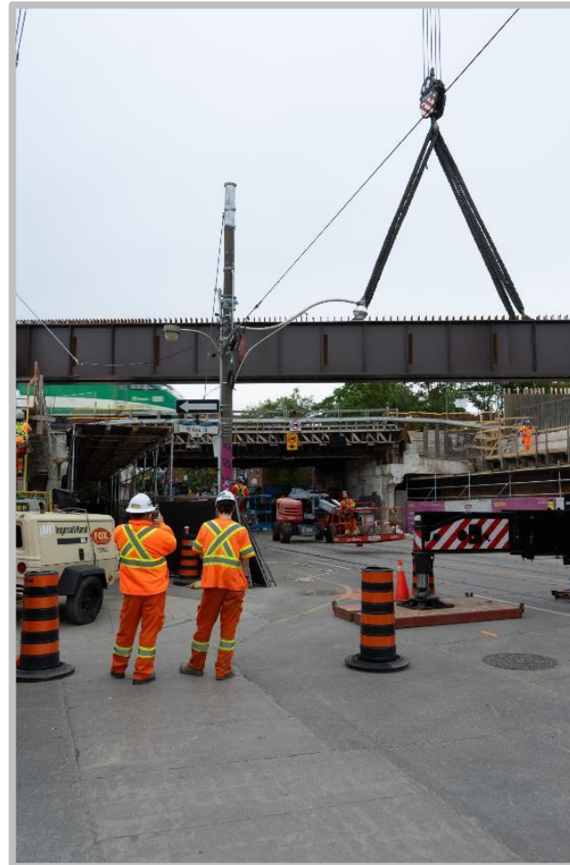
Installing the first girder for the new Queen Bridge
