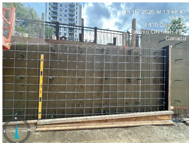
Dupont sidewalk wall reinforcement
