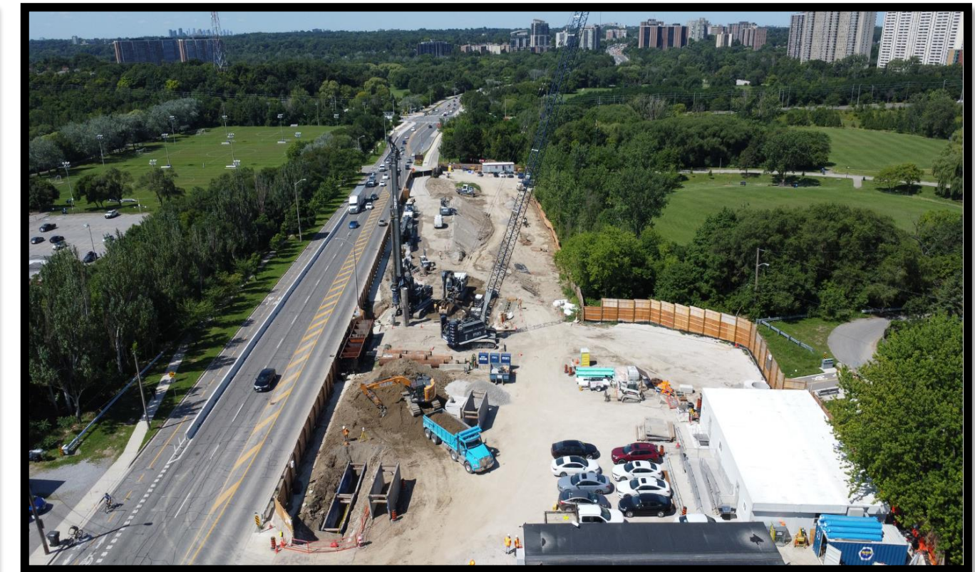
Drilling holes for excavation support
