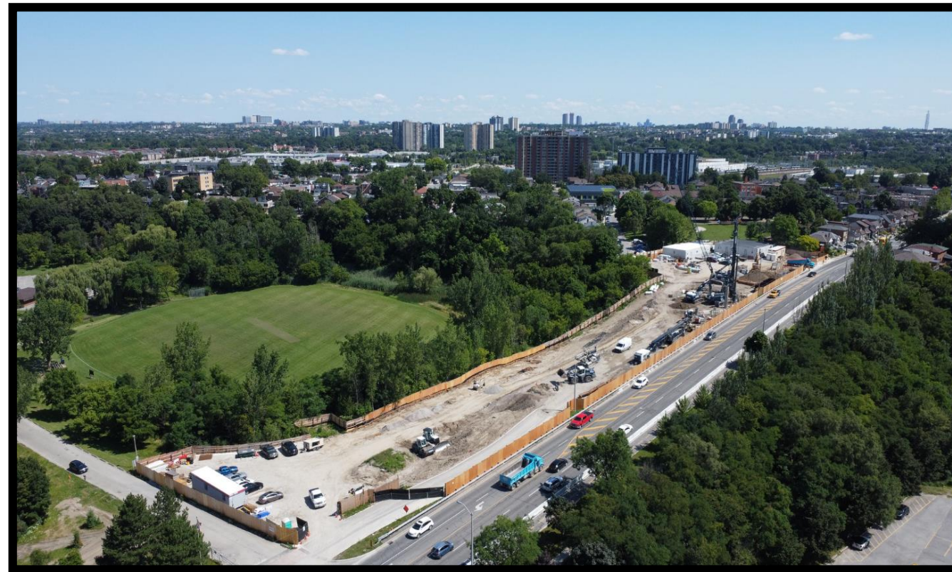
Preparation For excavation support
