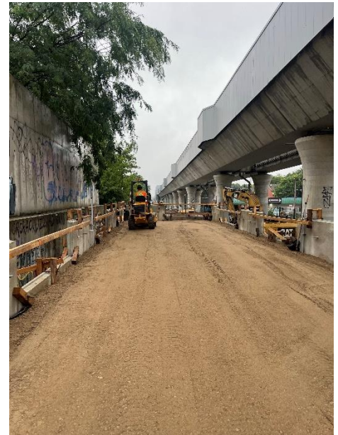
Completed more than 50% of the new switchback ramp structure
