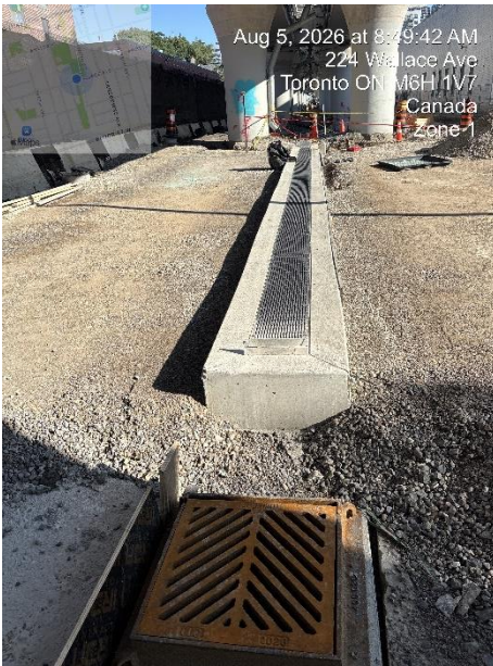
Completed trench drain installation at north Wallace
