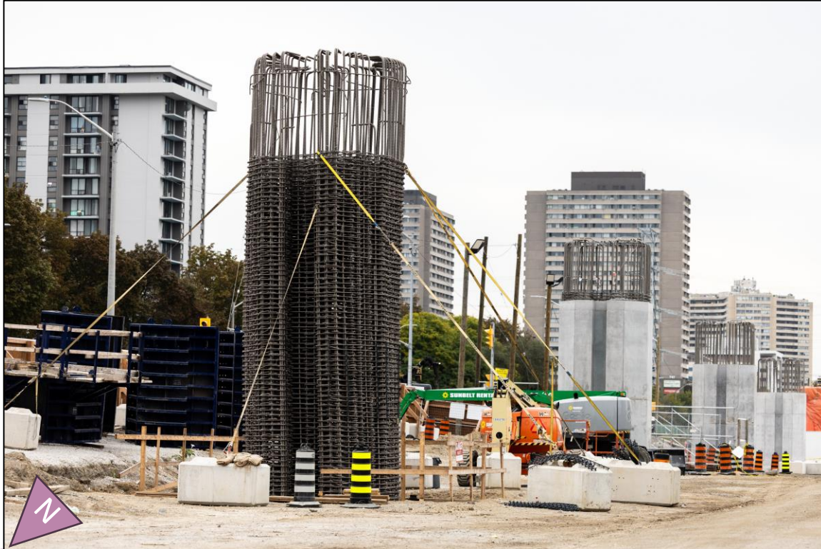
Rebar installation at D-23 , September 30, 2026
