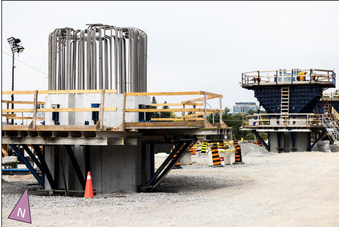
Column for pier at D-43, Sept. 30, 2026
