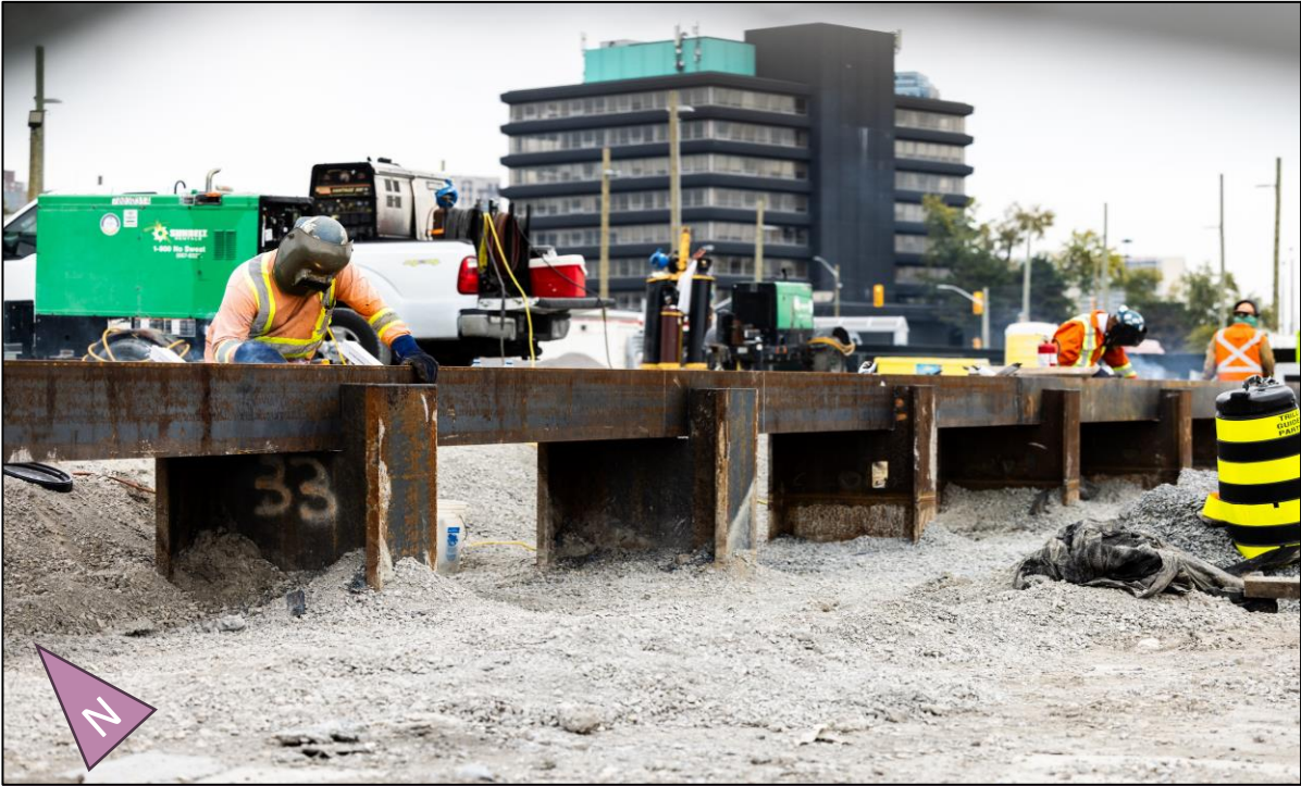
Welding steel beams for south wall, September 30, 2026
