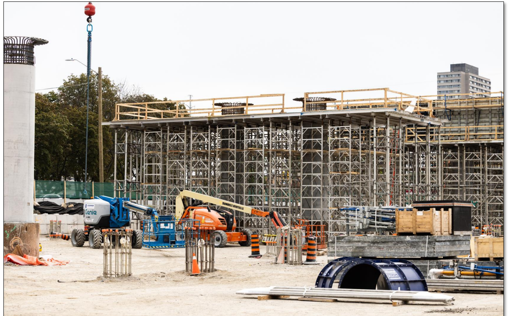
Scaffold installation for pier cap construction at Piers D-12, September 30, 2026
