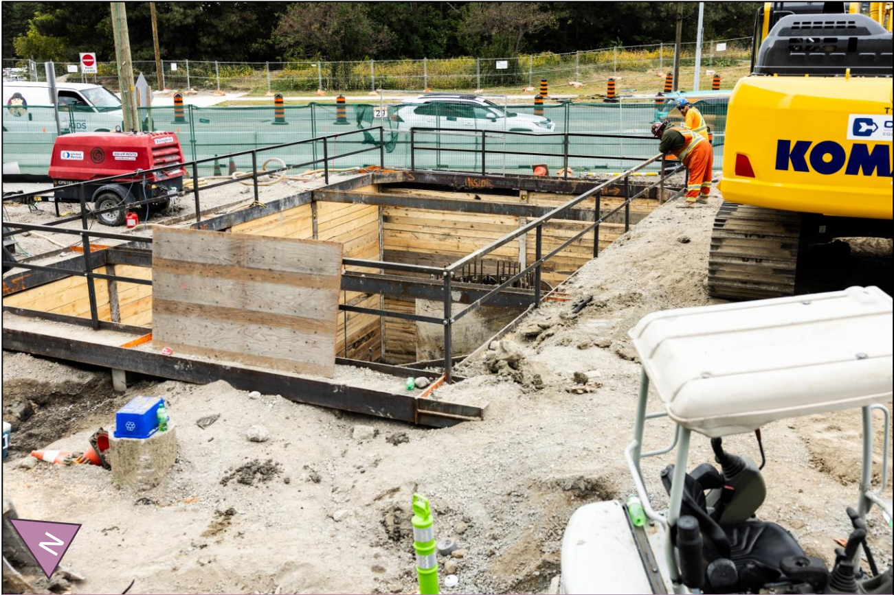
Pile cap work at D-27, September 30, 2026
