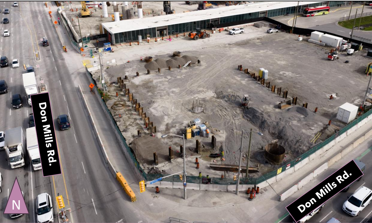
Don Mills Road and Eglinton Avenue East, September 9, 2026
