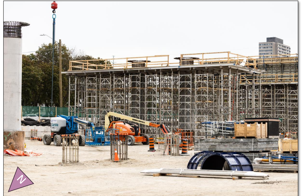
Scaffolding for Pier cap work at D-12 & D-10, September 30, 2026
