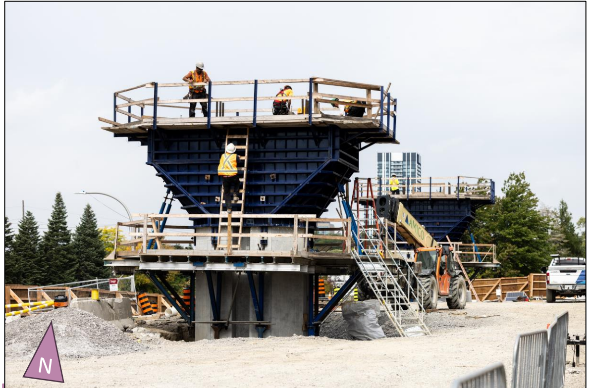
Pier cap forms at piers D-44 and D-45, Sept. 30, 2026
