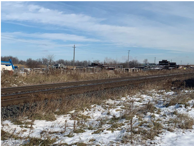
Figure 3-4: CN Works Yard just north of the Project Site.
