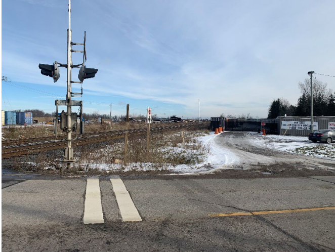
Figure 3-2: Self-storage facility and track crossing at Winston Churchill Blvd.
