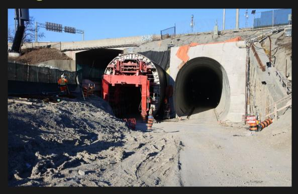
The cast in place tunnel liner is being prepared and moved into tunnel two to start the final liner installation.
